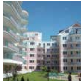
Location_Czech Republic Project_Apartment Building
